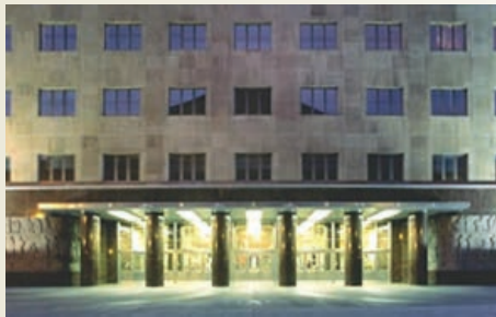
GAO headquarters building. Source: GAO Archives.
