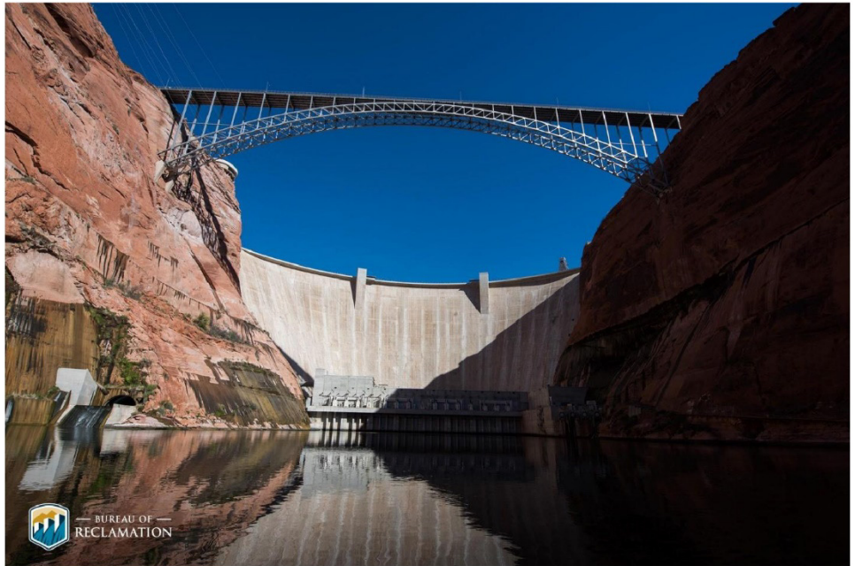
Figure 2: Photograph of a Dam
