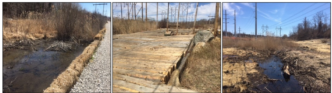
Access road in a wetland for a transmission line project
