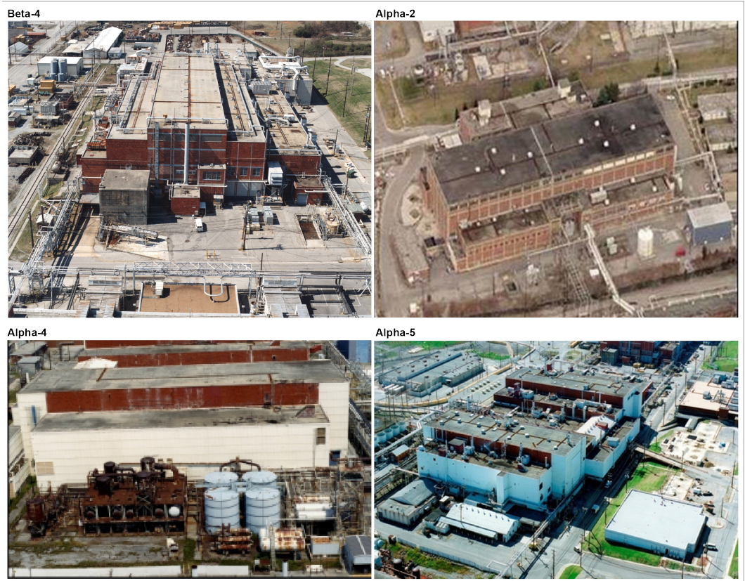
Source: U.S. Department of Energy (DOE) Office of Environmental Management – Oak Ridge. | GAO-24-107096
