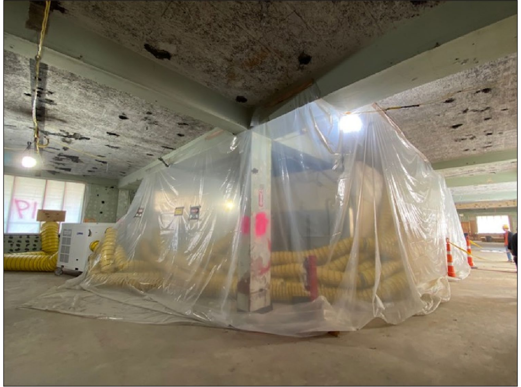
Figure 3: Samuels Hall Renovation Project, Which Includes the U.S. Merchant Marine Academy's Main Data Center, October 2023
