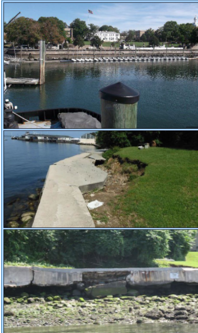
Figure 5: U.S. Merchant Marine Academy Seawall Repair and Rehabilitation Project
