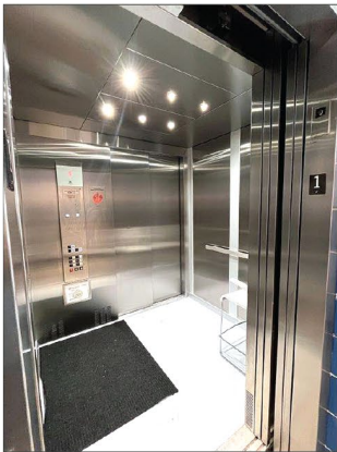
Elevator to help access living quarters above ground level.
