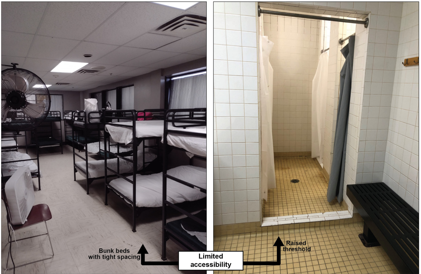
Figure 9: Example of a Shelter Room with Bunk Beds and Shower Area with a Raised Threshold
