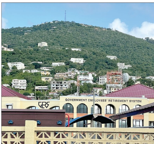
The GERS building is a three-story office complex of more than 68,000 square feet.
