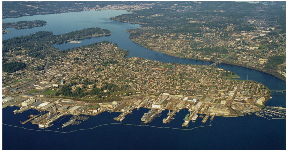
Figure 3: Puget Sound Naval Shipyard and Intermediate Maintenance Facility
