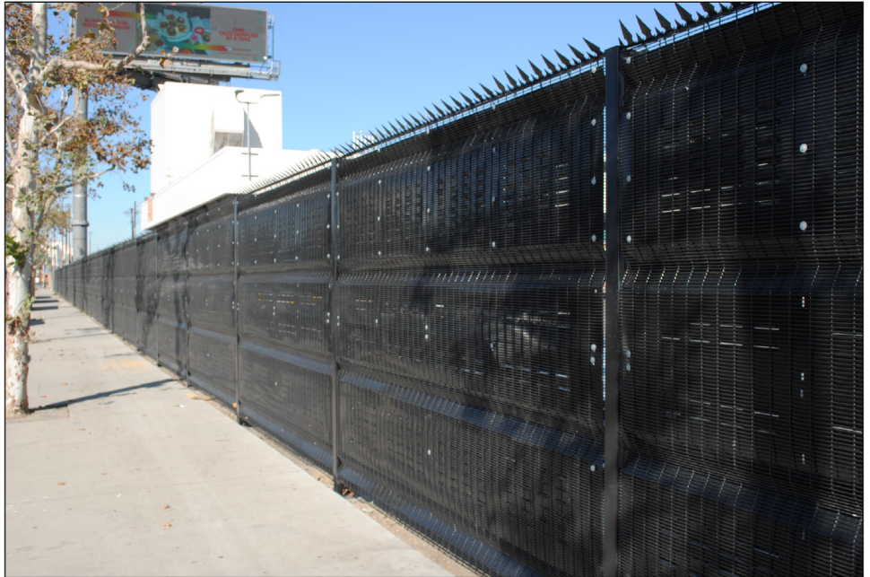
Figure 7: Fence Funded by the Transit Security Grant Program
