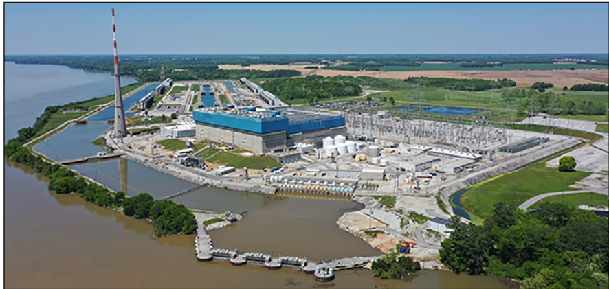
Tennessee Valley Authority's Browns Ferry Nuclear Plant in Alabama
