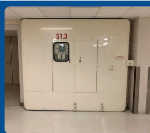
Watertight enclosure to prevent floodwater damage
