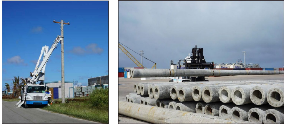
Figure 14: Concrete Utility Poles Installed in the Commonwealth of the Northern Mariana Islands as a Hazard Mitigation Initiative
