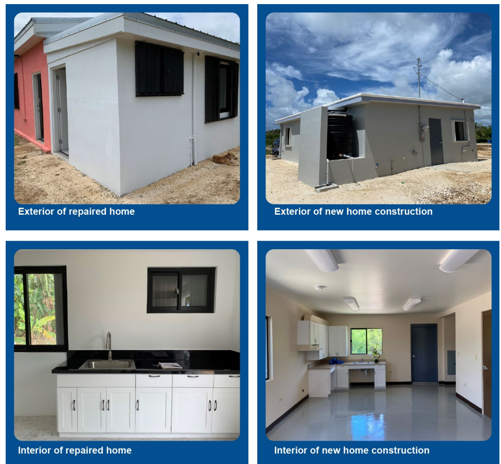
Figure 9: Completed Housing Repair and New Construction in the Commonwealth of the Northern Mariana Islands
