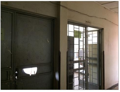
Figure 14: Damaged Exterior Door and Exposed Wiring at Bahir Dar Veterinary Lab in Ethiopia
