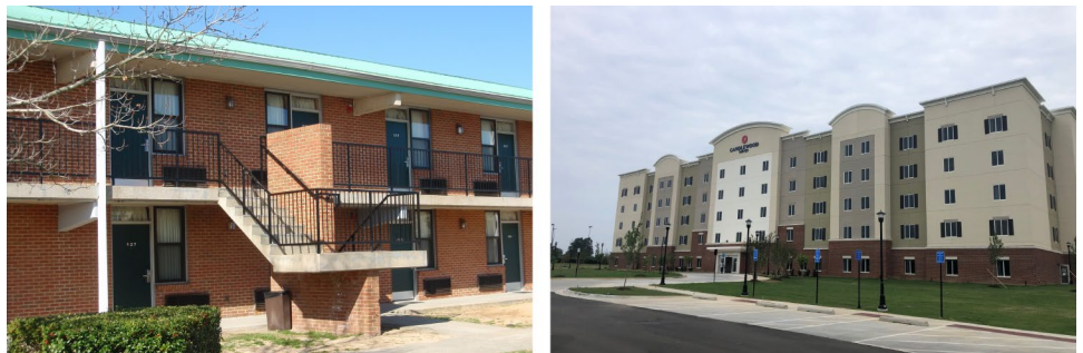
Figure 14: The Army Replaced Lodging at Fort Gordon, GA, with a Candlewood Suites Hotel in 2020 as Part of the Privatized Army Lodging Program
