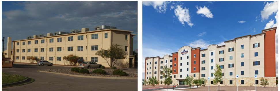
Figure 10: The Army Replaced Lodging at Fort Bliss, TX, in 2018 with a Candlewood Suites Hotel as Part of the Privatized Army Lodging Program
