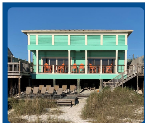
Structure elevation to mitigate flood damage
