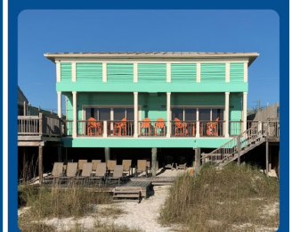
Structure elevation to mitigate flood damage
