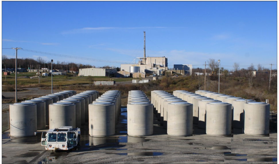
Figure 4: High-Level Waste from the West Valley Demonstration Project in Interim On-Site Storage, March 2017
