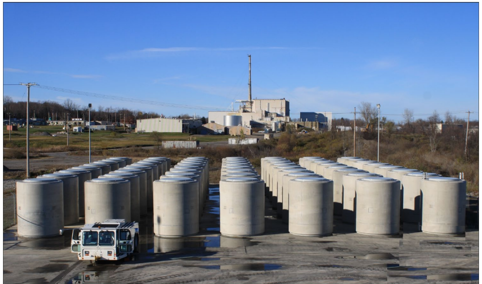
High-Level Waste from the West Valley Demonstration Project in Interim On-Site Storage, March 2017
