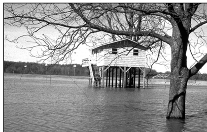
Example 1: Building elevated on piers
