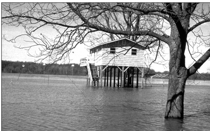
Example 1: Building elevated on piers
