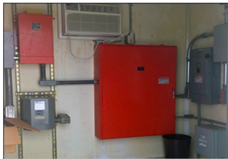
A shack that houses a medium-intensity approach lighting system with sequenced flashers at the Charles B. Wheeler Downtown Airport in Kansas City, Missouri
