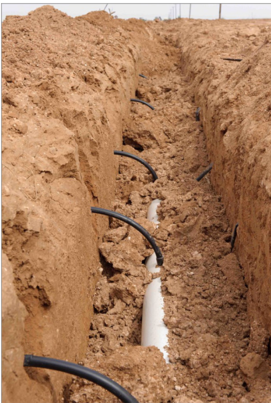
Figure 12: Subsurface drip irrigation
