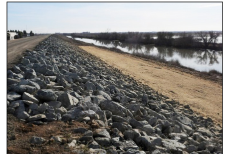
Completed in 2009, the U.S. Army Corps of Engineers rebuilt and added rip rap, or large rock, to the waterside banks of a 400-foot stretch of levee near the Yolo Bypass in West Sacramento, CA.
