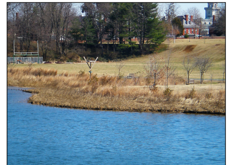
The living shoreline uses marsh plants and other natural features to protect the shore from erosion.
