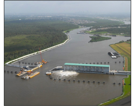
New Orleans' Hurricane and Storm Damage Risk Reduction System is comprised of numerous features including levees, floodwalls, floodgates, surge barriers and pump stations.
