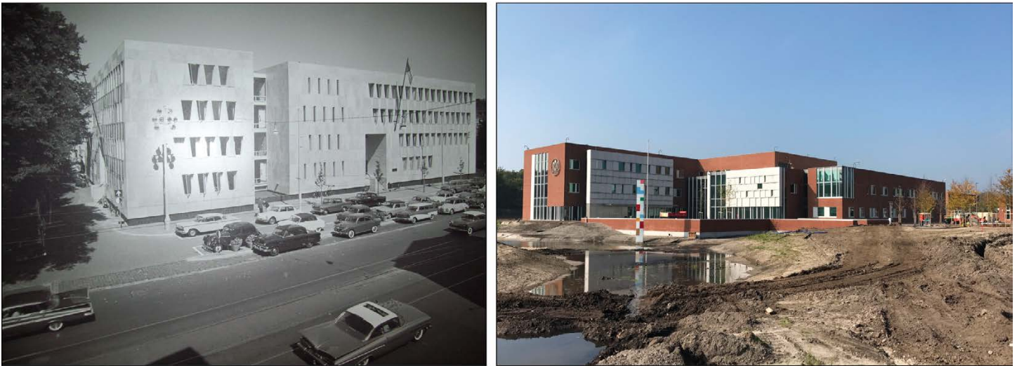
Figure 20: U.S. Embassy, The Hague, Netherlands: Former U.S. Embassy, Built in 1959 (Historical Photo), the New U.S. Embassy under Construction, and Timeline
