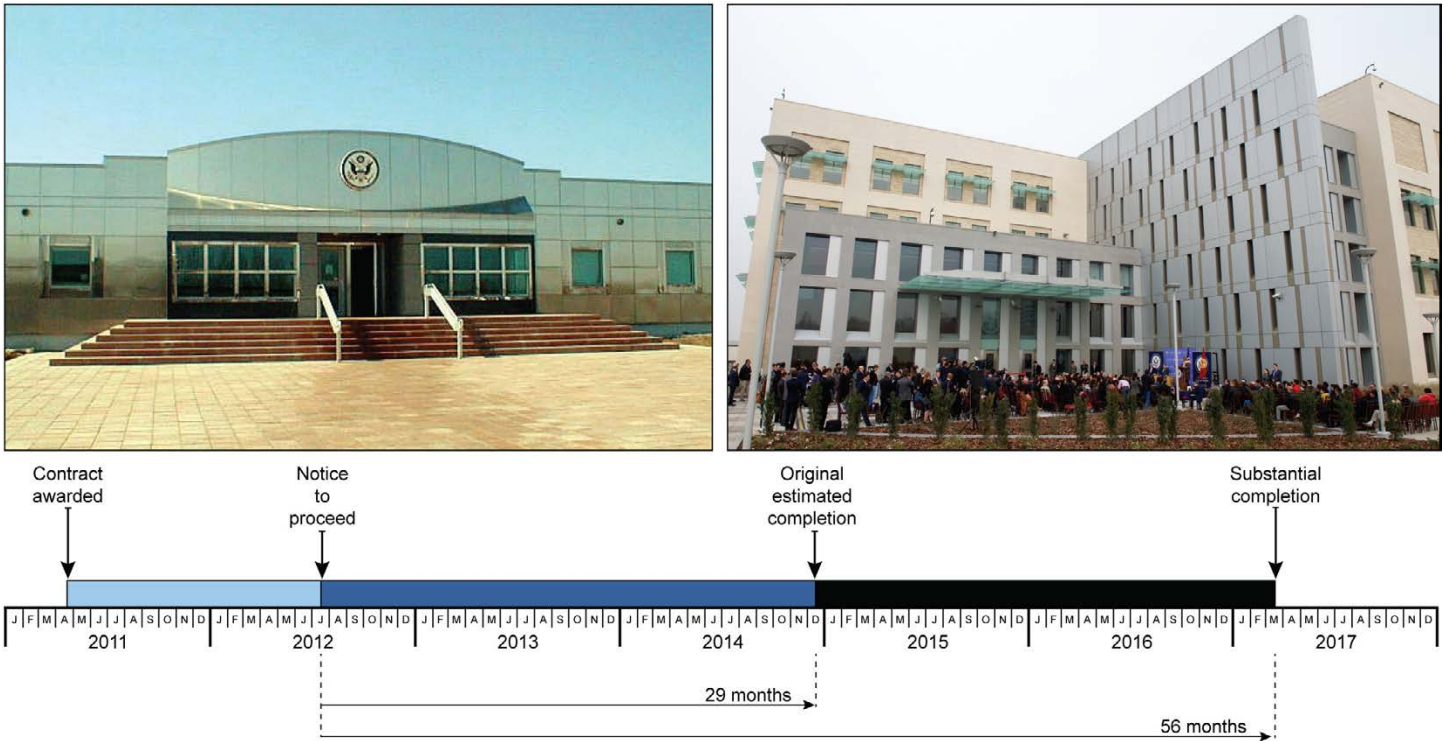
Figure 17: U.S. Embassy in Bishkek, Kyrgyzstan: Original Chancery Office Building, New Chancery Office Building, and Timeline
