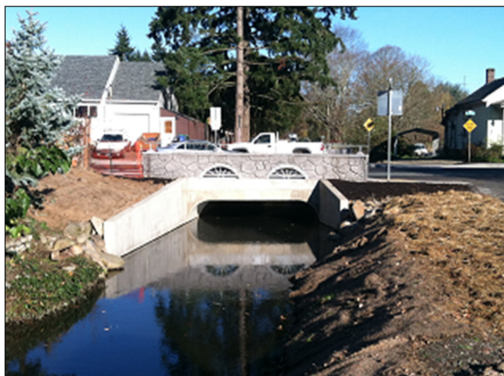
Figure 6: Before and After Pictures of Tacoma Street Culvert Replacement in Portland, Oregon
