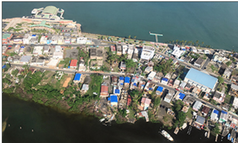
Damaged buildings with temporary roofing, Puerto Rico.
