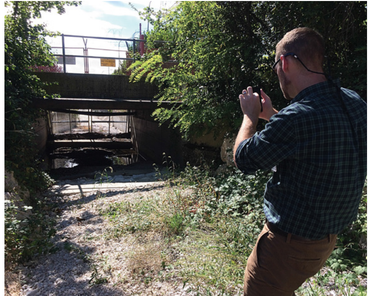
Analyst documents structure damage at Aviano AFB, Italy during a review of overseas climate change adaptation.
