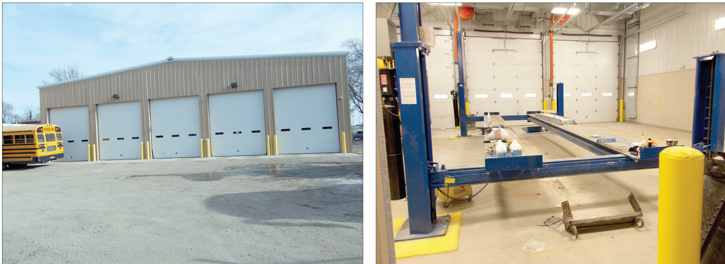
Figure 7: Exterior and Interior of Recently-Constructed School Bus Maintenance Building Where Door Does Not Close When a Large School Bus Is On Hydraulic Lift
