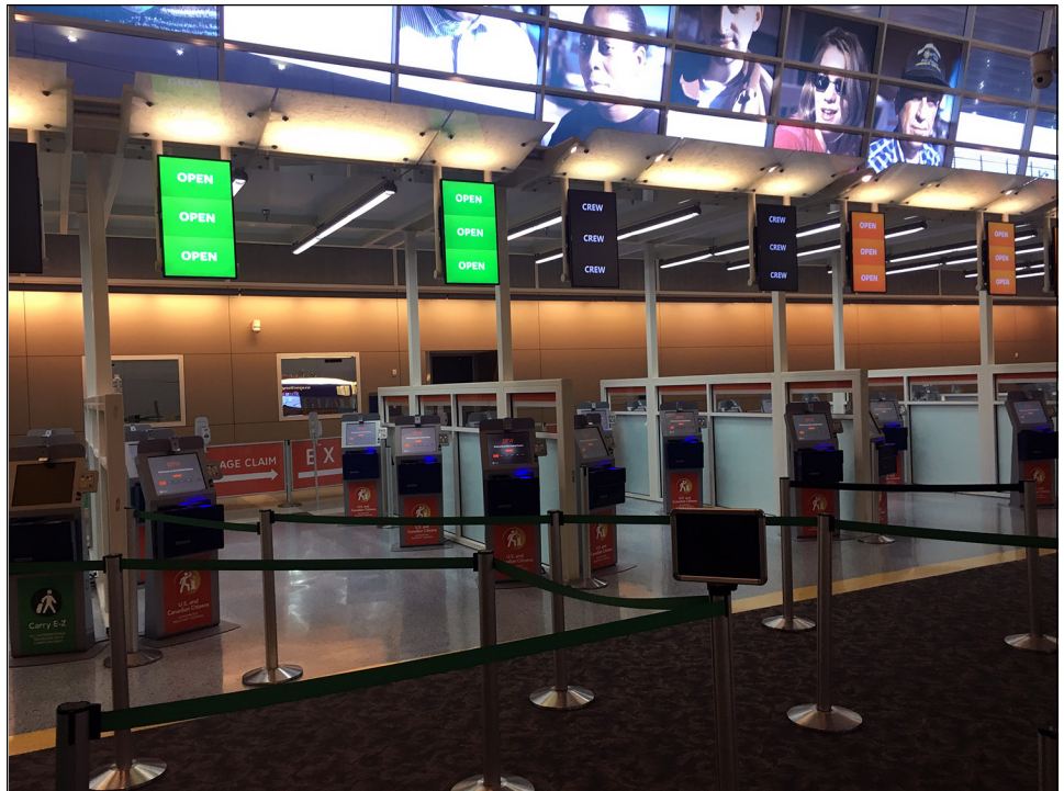
Figure 41: Variable Message Signage Above Automated Passport Control (APC) Kiosks at Dallas/Fort Worth International Airport (DFW)
