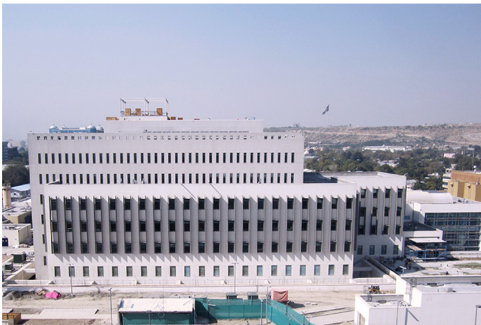
Figure 4: U.S. Embassy Kabul, West Compound, Office Annex A
