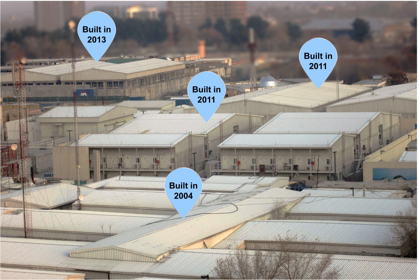
Figure 7: U.S. Embassy Kabul, Temporary Facilities
