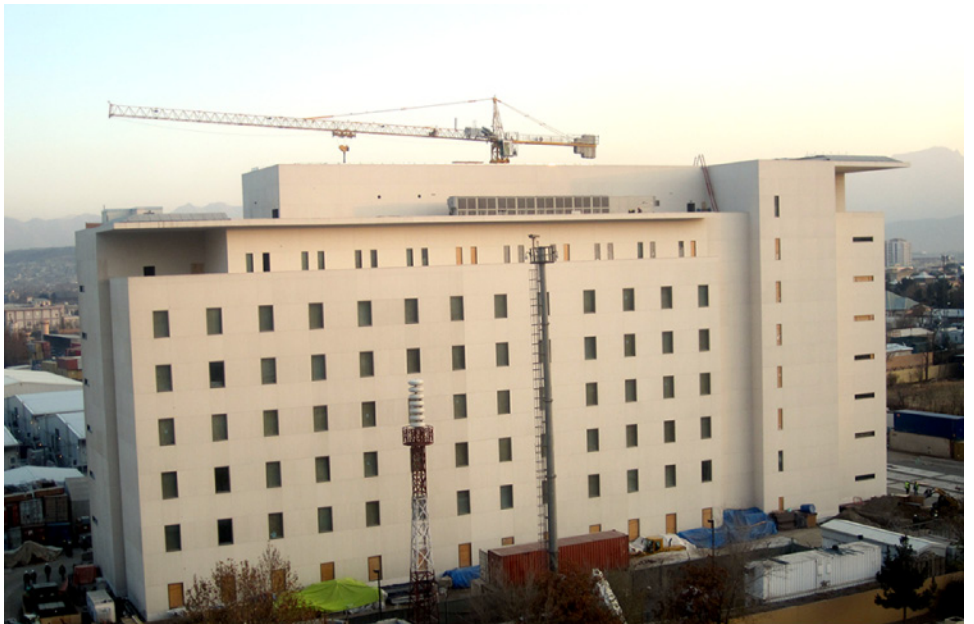
Figure 6: U.S. Embassy Kabul, East Compound, Apartment Building 1
