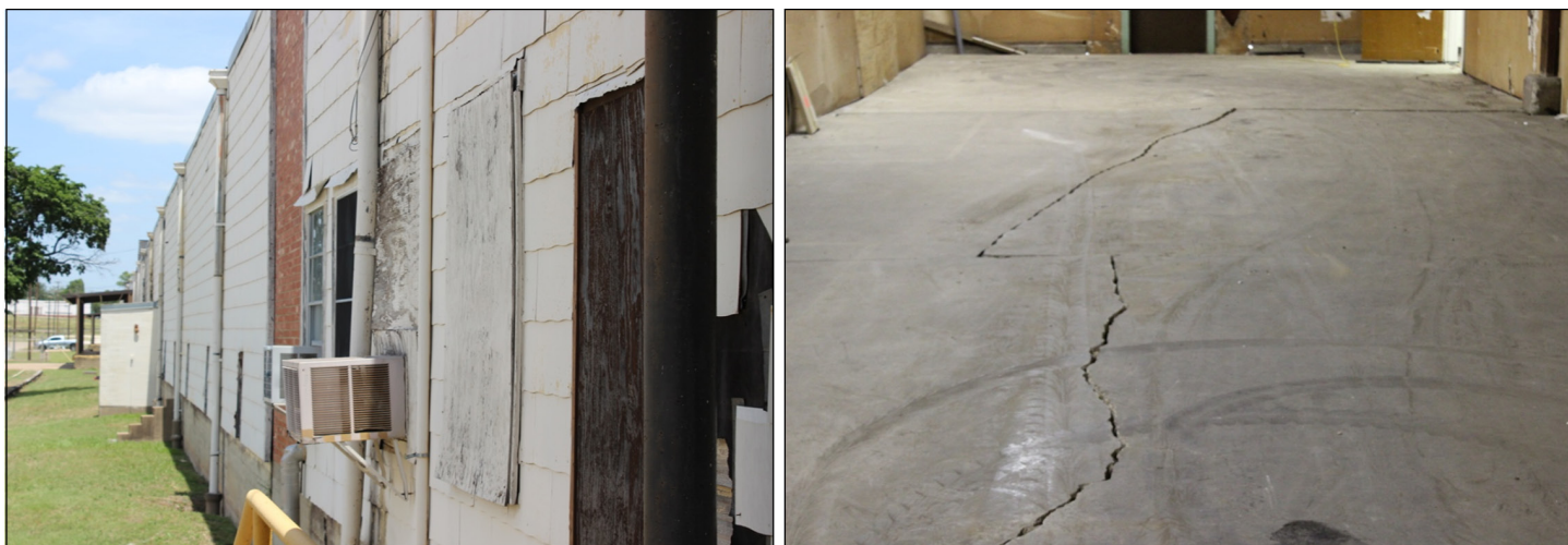
Figure 5: Aging Occupied GSA Warehouse in Ft. Worth, Texas
