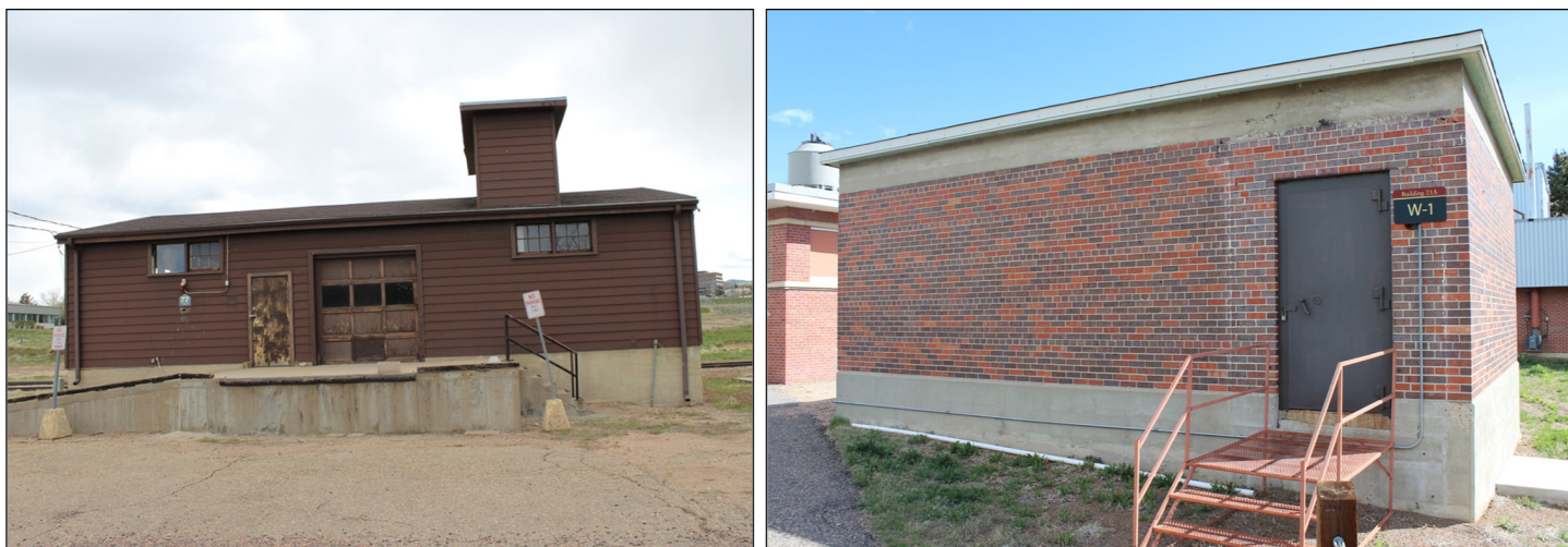
Figure 6: GSA Held Warehouses in Lakewood, Colorado, Pending Historic Designation
