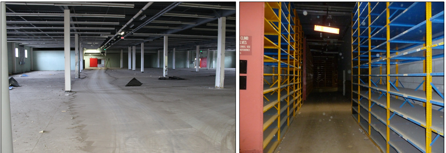
Figure 7: Vacant GSA Warehouse Formerly Used by the National Archives and Records Administration, Lakewood, Colorado
