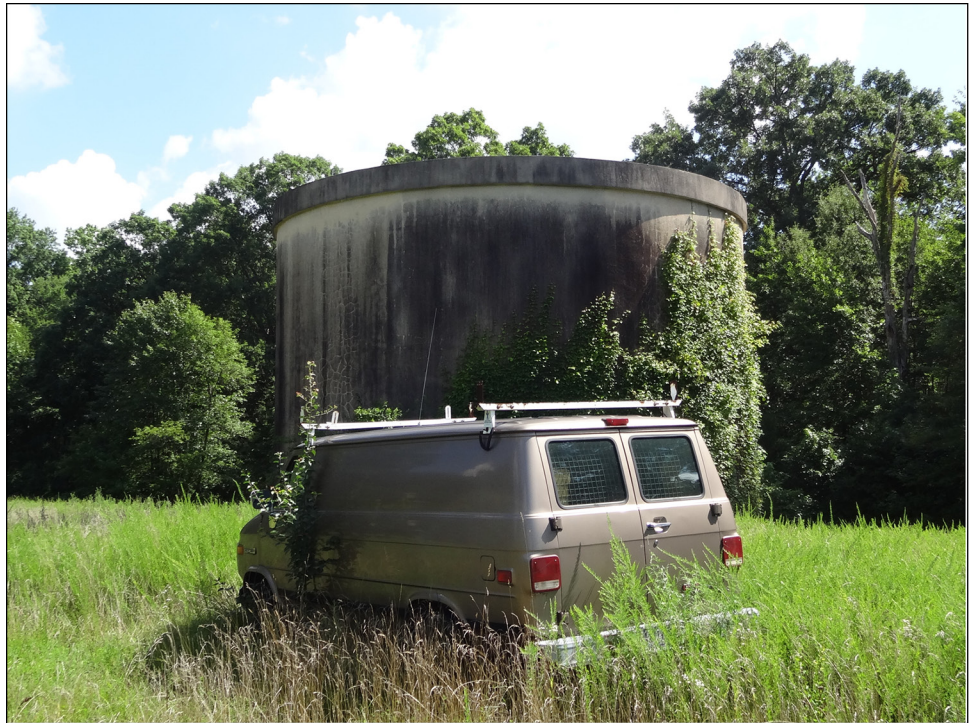
Figure 10: Unused Water Tower at USDA's Beltsville Facility, Maryland
