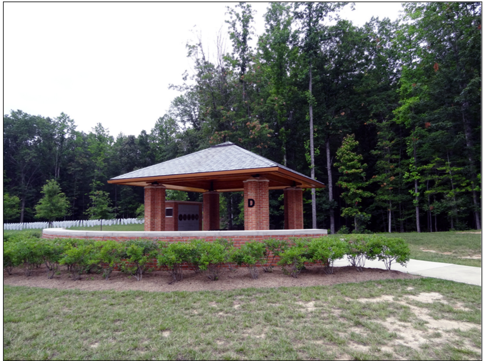
Figure 6: Example of Zero Annual Operating Costs for a Structure, a Committal Shelter at Quantico (VA) National Cemetery, Virginia
