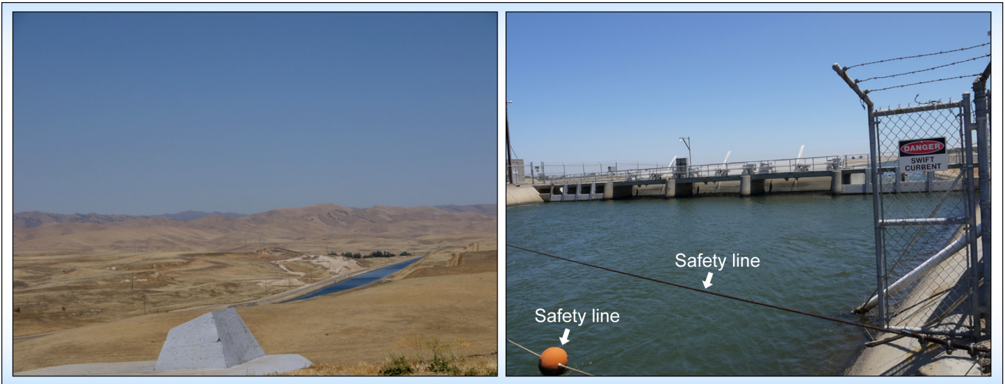
Figure 9: Examples of Security and Safety Challenges Presented by the Long Length of and the Swiftly Flowing Water in the Delta-Mendota Canal in California
