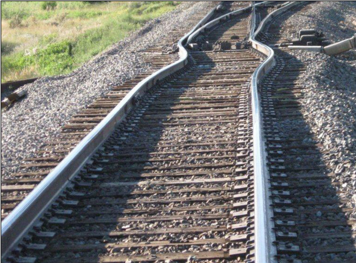
Example of excessive heat forcing the rails out of alignment
