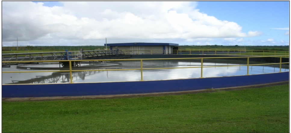
Figure 4: Northern District Wastewater Treatment Plant
