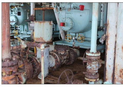
Figure 1: Corrosion on Platform Hogan in the Pacific Region
