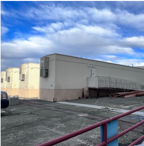
External modular units housing the mammogram machine, bone density scanner, and other departments.
