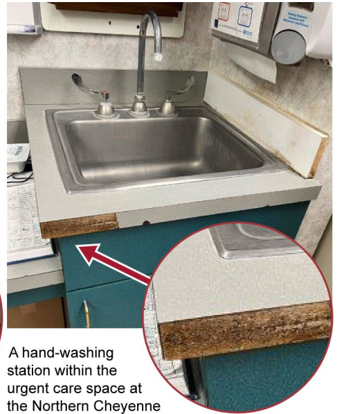
Figure 7: Examples of Deteriorating Building Components: Rusted Cabinet, Damaged Countertop, and Missing Flooring from Selected Site Visits
