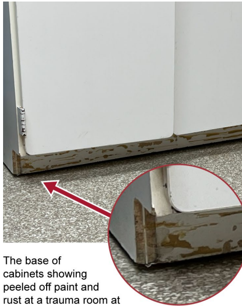
Figure 7: Examples of Deteriorating Building Components: Rusted Cabinet, Damaged Countertop, and Missing Flooring from Selected Site Visits
