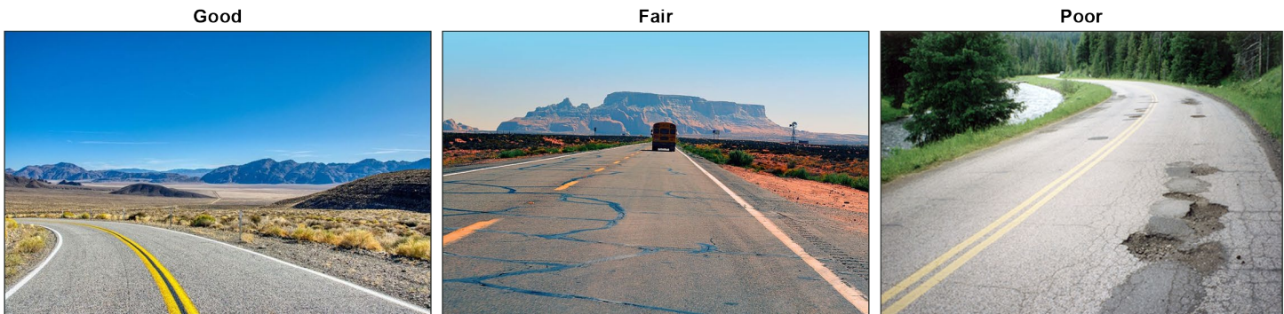
Figure 4: Illustrative Examples of National Highway System Pavement Sections in “Good,” “Fair,” and “Poor” Condition, as Categorized by the Federal Highway Administration
