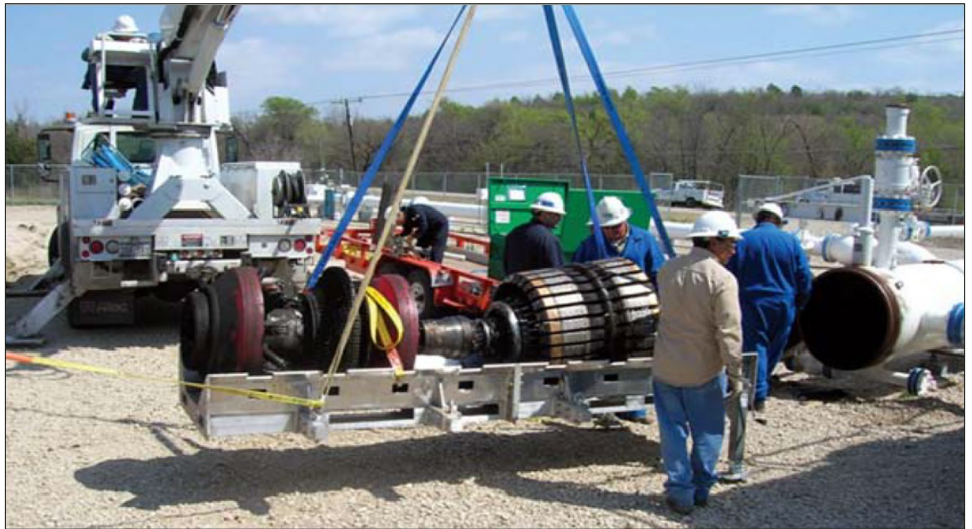
Figure 2: In-Line Inspection Tool Being Placed in a Launch Point on a Pipeline
