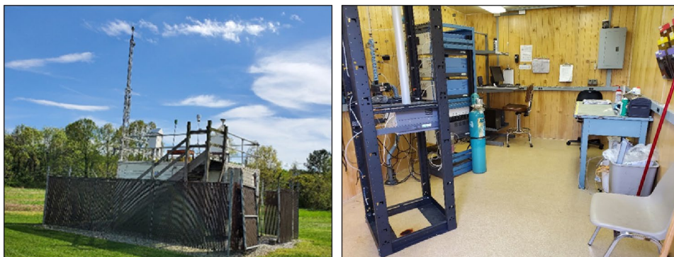
Exterior and interior of a monitoring site that is over 30 years old operated by the Delaware Department of Natural Resources and Environmental Control
