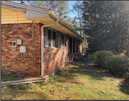
Exterior showing bushes and trees trimmed away from the walls and gutters.
