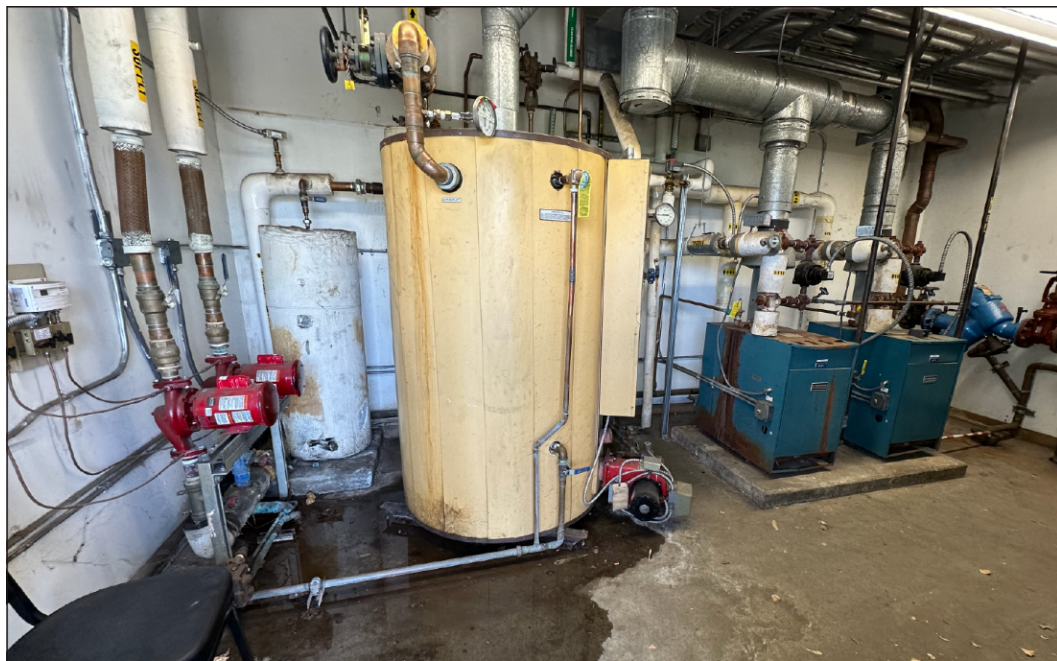
Figure 8: Example of Coast Guard Maintenance Project
