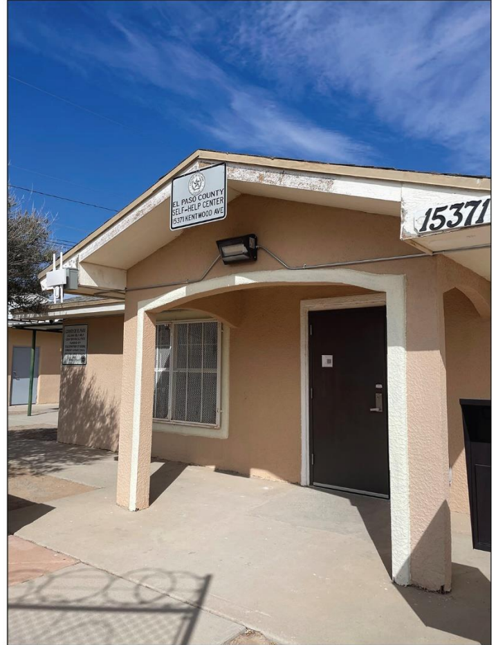
The El Paso County Self-Help Center, which serves five colonias in El Paso County, Texas.
