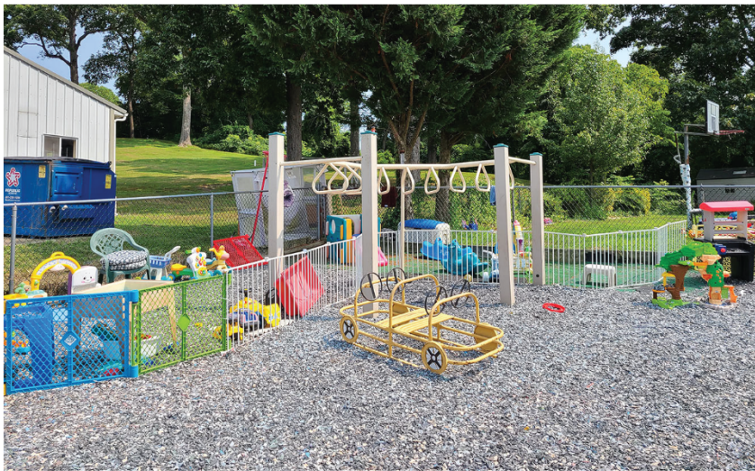
Uneven surfaces in and around playgrounds limit access for children in wheelchairs
