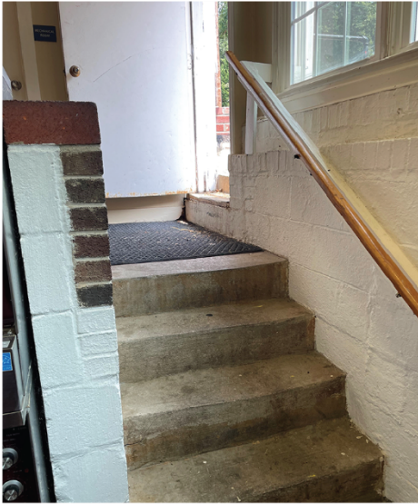
Stairs leading to multipurpose room
