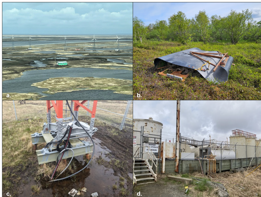
a. Aerial view of wind turbines supplying power to a microgrid in a remote Alaska Native village. b. Sled used to pull wind turbine components over the tundra to be assembled for a microgrid in a remote Alaska Native village. c. Base of a wind turbine in a remote Alaska Native village that is no longer flush with the ground due to thawing permafrost. d. Aging bulk fuel storage infrastructure in a remote Alaska Native village.
