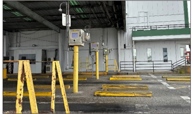
RFID and OCR technologies at SSA Marine Pacific Terminal in Long Beach.
