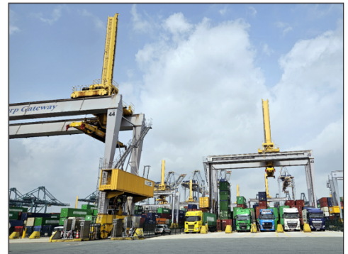
Automated rail-mounted gantry cranes at DP World Antwerp Gateway in Antwerp, Belgium.
