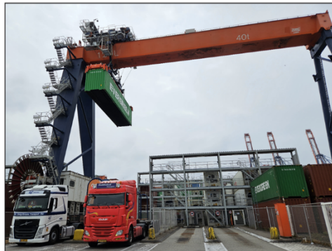
Automated rail-mounted gantry cranes at Hutchison Ports ECT Euromax in Rotterdam, The Netherlands.
