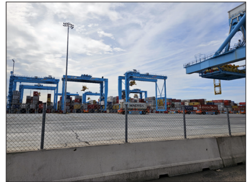
The automated area of the terminal (the yard) is fenced off from areas with workers, reducing the potential for injuries.
