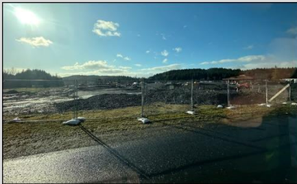
Kodiak Family Housing construction site.
