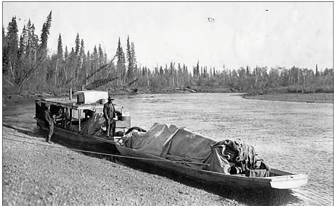
Figure 3: Photograph Showing Historical Use of Waterway for Travel for Commerce
