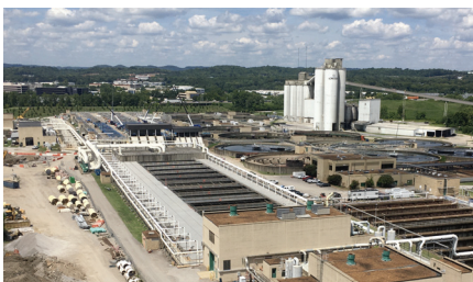
Central Wastewater Treatment Plant Capacity Improvements Project Source: Metro Water Services. | GAO-23-105285
