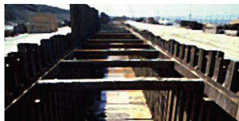
Construction of Westside Transport/Storage Structure
