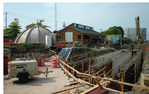
Excess Flow Management Facility Upgrade Source: City of Oswego, New York. | GAO-23-105285
