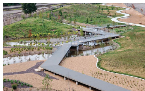
Central Industrial District Green Infrastructure Project in the Turkey Creek Watershed to manage stormwater and reduce CSOs. Source: KC Water. | GAO-23-105285
