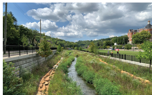
Lick Run Project in Cincinnati, Ohio, summer 2022 Source: Metropolitan Sewer District of Greater Cincinnati. | GAO-23-105285
