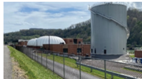
Star City Wastewater Treatment Plant Source: GAO photo. | GAO-23-105285
