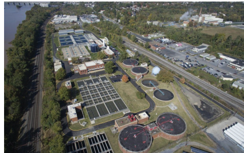
Capital Region Water's Advanced Wastewater Treatment Facility Source: Capital Region Water. | GAO-23-105285
