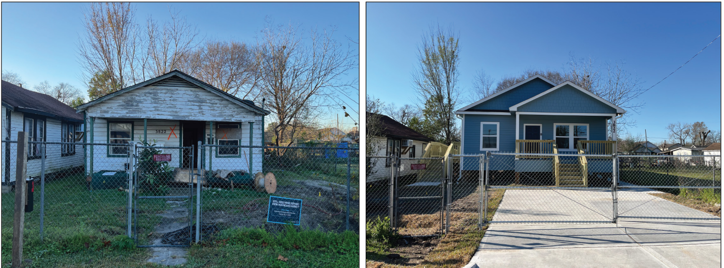
Figure 6: Pictures of a Home Repaired under Texas’s Homeowner Assistance Program
