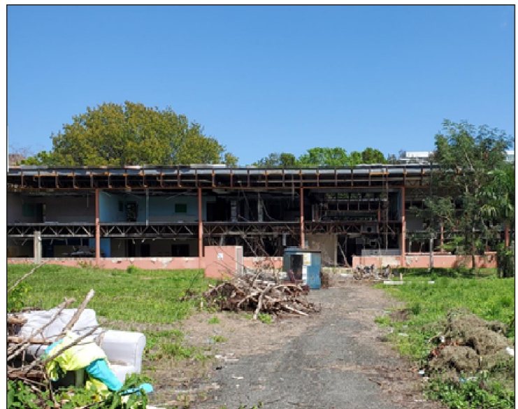
School observed in March 2022 awaiting repairs. According to a FEMA official, a construction crew removed doors, windows, and some walls due to asbestos and lead in the building.
