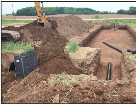
Bioreactor being built
