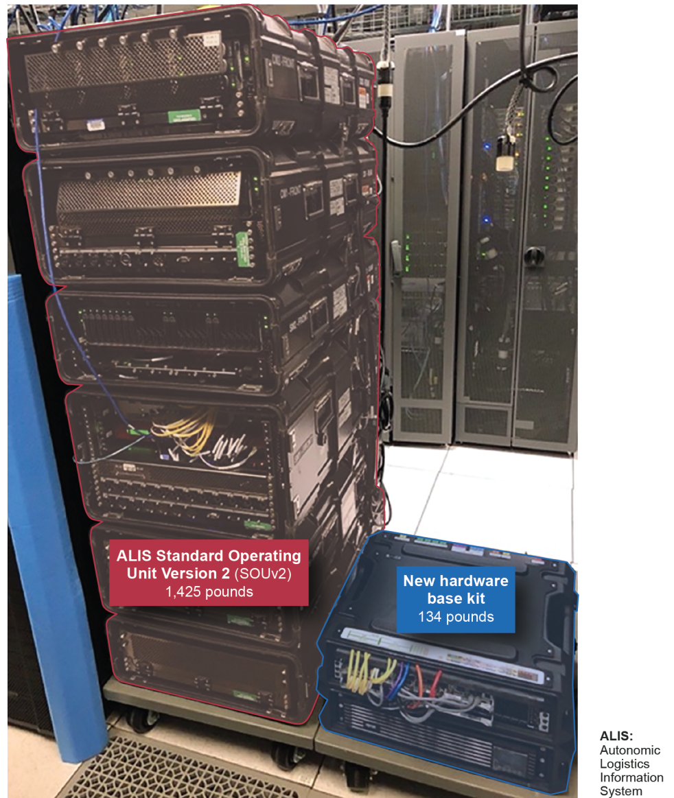
Figure 12: New Hardware Is Smaller than ALIS Hardware
